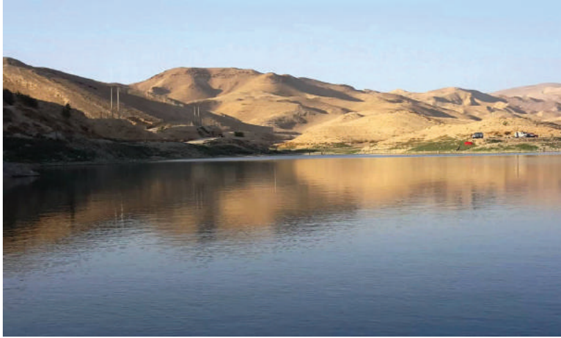
Al-Kafreen Dam (Metal Works)
